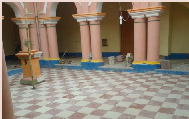
Neue Fliesen in Jamdaha!
